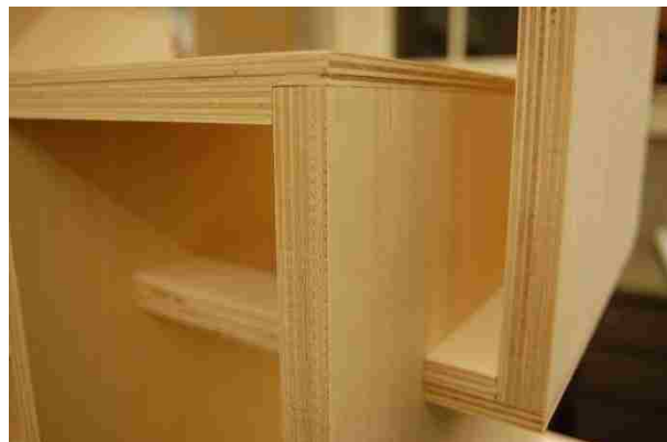
Fig. 9.7 Intersecting and emerging joinery conditions
